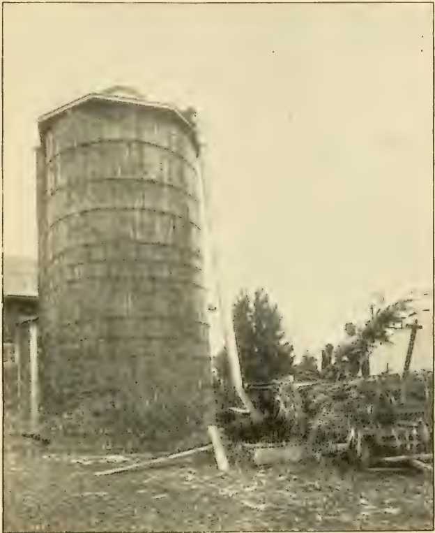
Fig 43—Filling Silo with Blower
